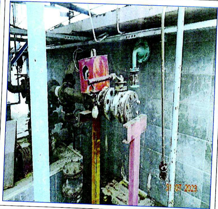
Marine line disconnection After photographs
