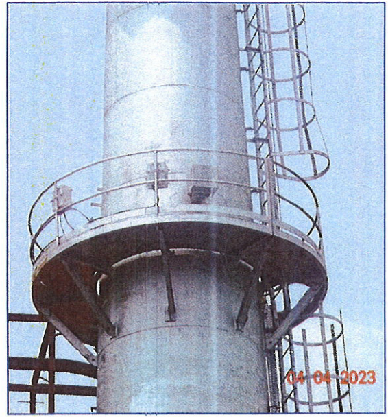
CEMS provided to 16 TPH Boiler
