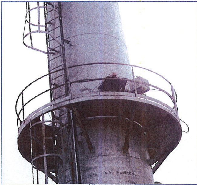
CEMS provided to 16 TPH Boiler
